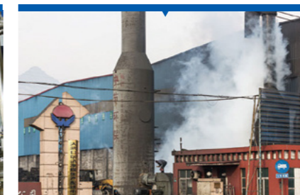
煤化工行业 Coal chemical industry
