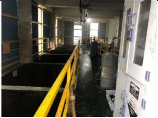
废液暂存仓围堰
