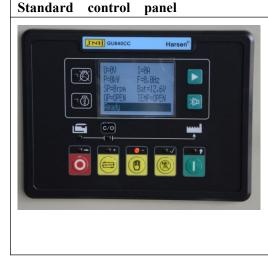
Standard control panel can satisfy the Genset for normal operation, it have the advantages of simple operation, multiple functions, reliable protection. The panel can receive remote open/stop control signal for Genset. (ATS control)
