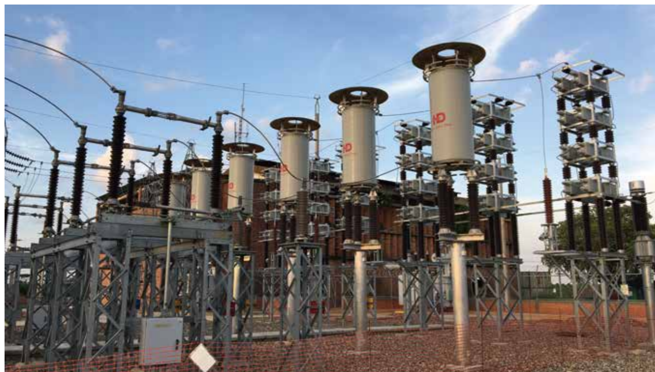
115kV DRY-TYPE AIR-CORE DAMPING REACTOR (COLUMBIA TIBU)
