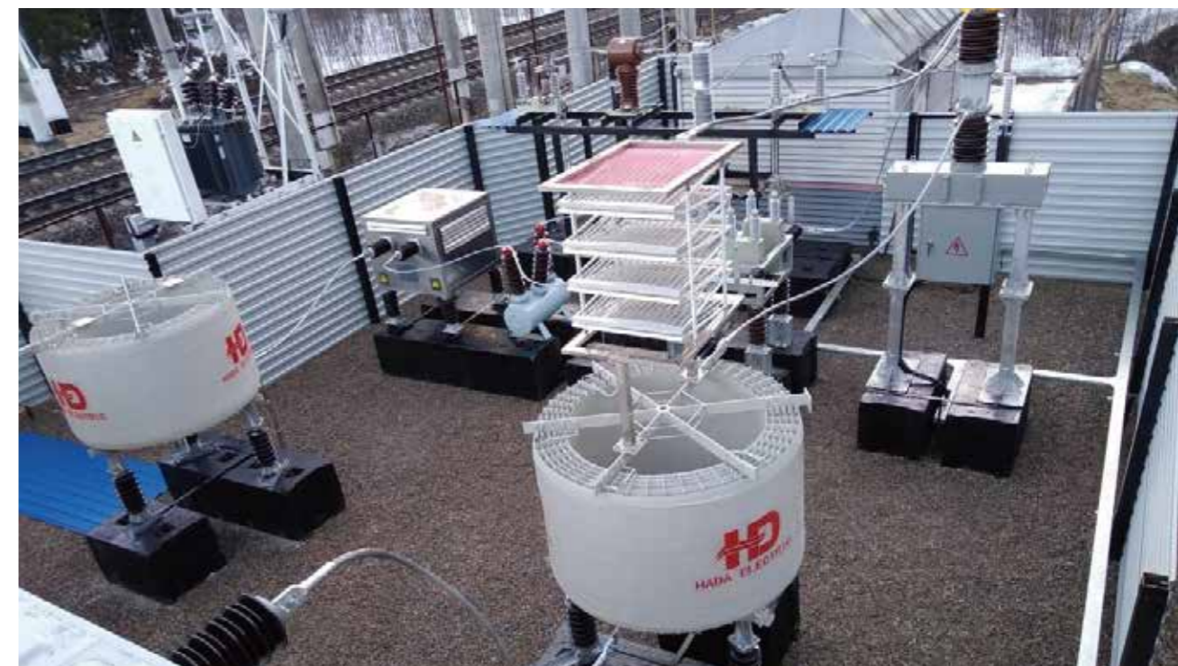
27.5 kV DAMPING REACTOR FOR ELECTRICAL RAILWAY(RUSSIA)
