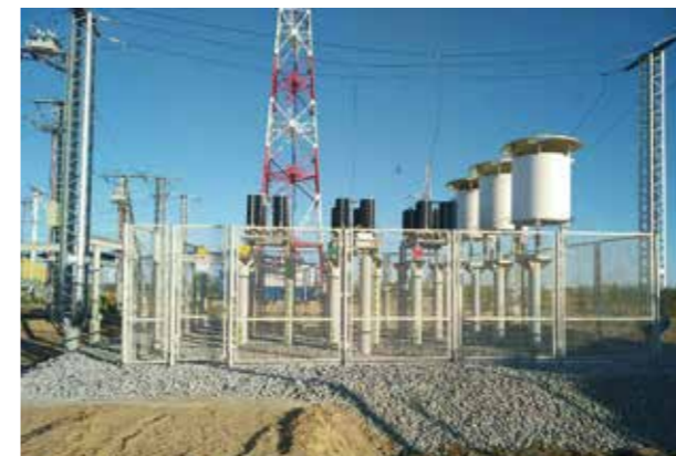
35kV SHUNT REACTOR (RUSSIA)
