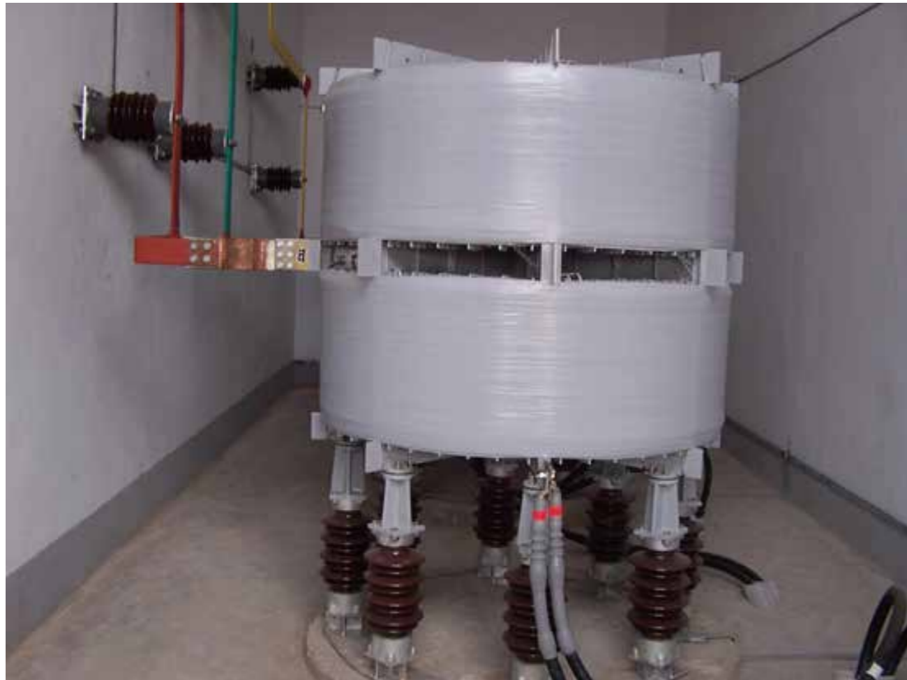
35kV DUPLEX CURRENT-LIMITING REACTORS (CHINA)
