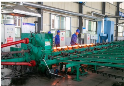
Finishing Mill Unit
