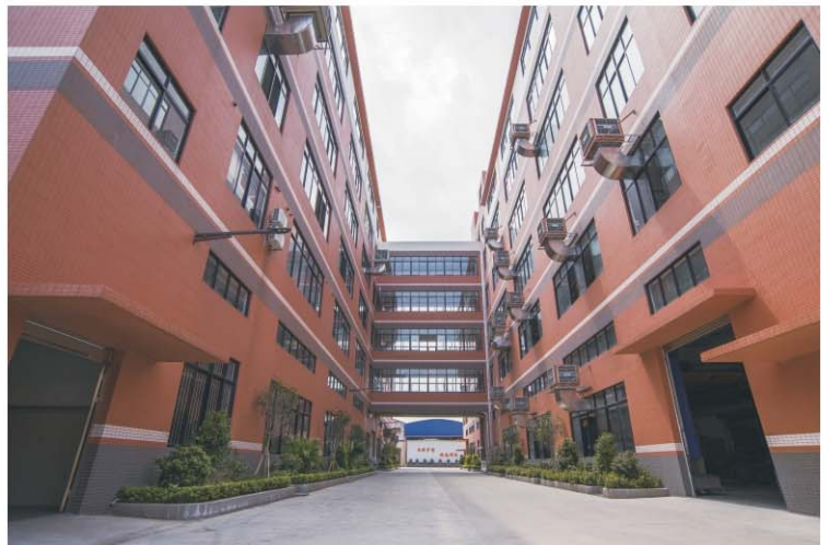
威浦局部厂区 Workshop building
