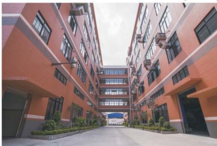
威浦局部厂区 Workshop building
