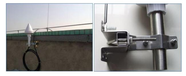
GNSS antennas can be installed on the edge of guardrail where no building more than 3mhigher than antennas is visible outside 10m around the antenna. Lightening protection measures for antennas. Outdoor antennas are generally installed within the lightning protection zone of the building. Arrester should be set up additionally if the antennas are higher or beyond the lightening protection zone. The arrester is as shown in the figure below.
