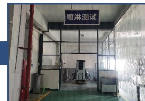
喷淋测试 Spray testing
